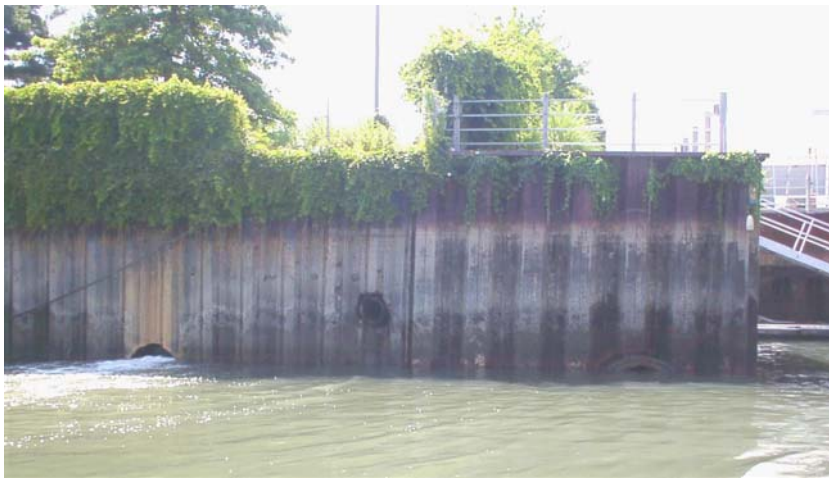
Glen Cove STP discharge (left); other outfall pipes
